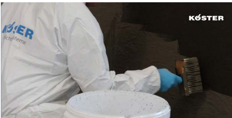
KÖSTER KD 1 Base: in 2 coats (second layer after 30 minutes)
